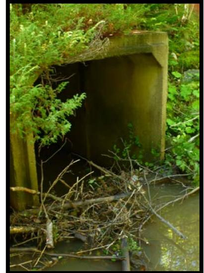
*Improper maintenance can cause culverts to become barriers to fish passage*
