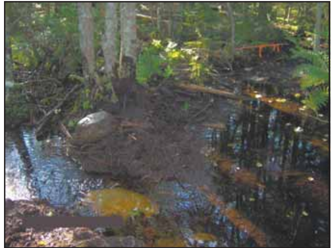
Dam after being open
